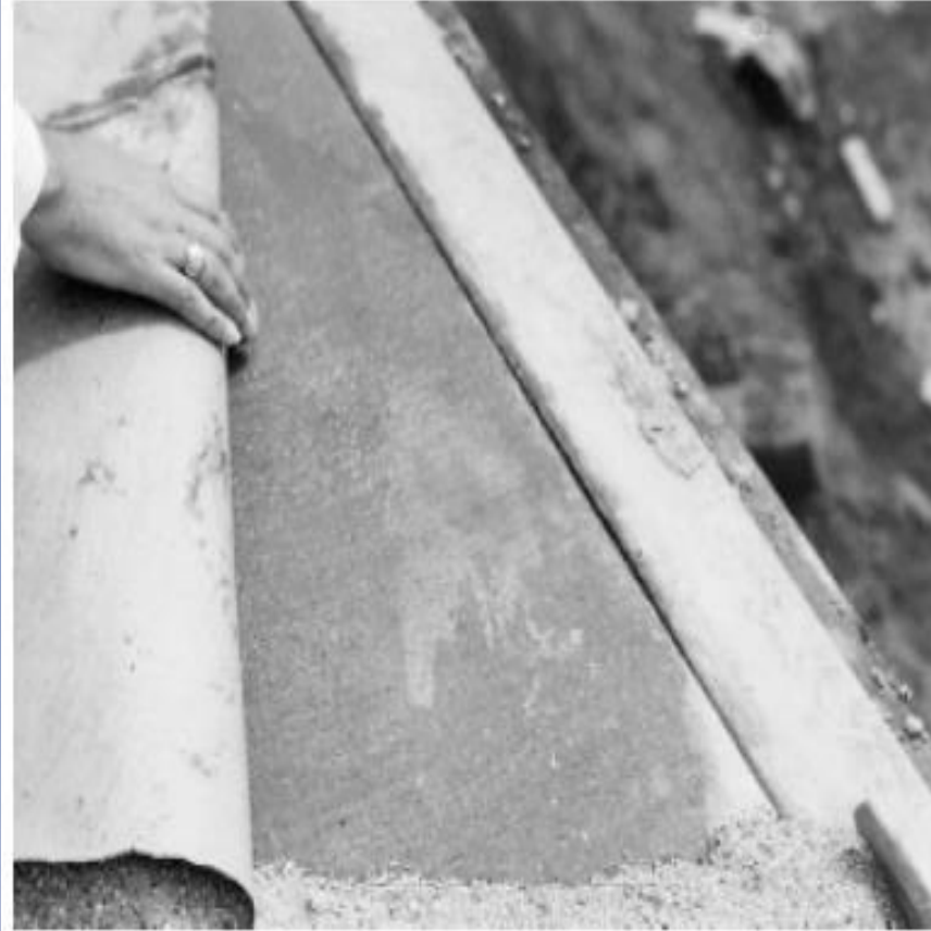
Fig.12-6. Impervious curing paper is an efficient means of curing horizontal surfaces. (IMG12361)
