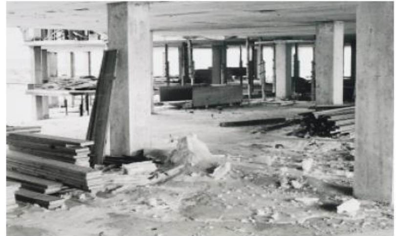
Fig. 14-11. Example of a concrete floor that was saturated with rain, snow, or water and then frozen, showing the need for air entrainment. (IMG12353)
