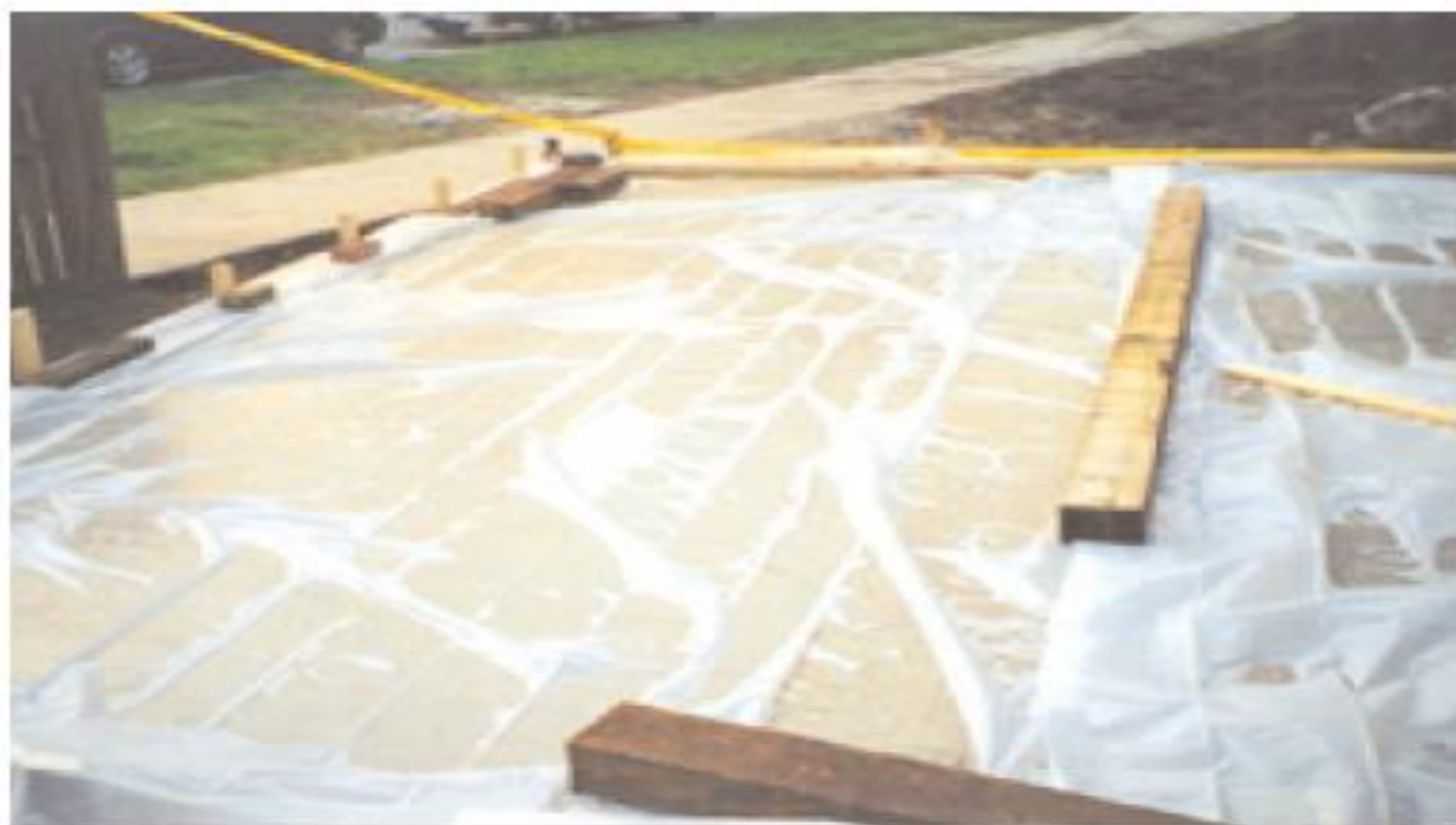
Fig. 12-7. Polyethylene film is an effective moisture barrier for curing concrete and easily applied to complex as well as simple shapes. To minimize discolouration, the film should be kept as flat as possible on the concrete surface. (IMG12360)
